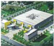
PLATE-FIN HEAT EXCHANGER SUB-FACTORY
